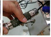
三通閥與進出水控制盒電源線連接 Connecting auto three way valve to controller.
