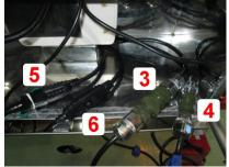
請將三通閥控制器電源線插入電源孔 Power the chilling water switch controller.
