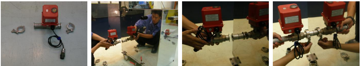
二通閥與進出水控制盒電源線連接 auto two way valve and controller wire connection.
