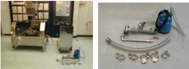
儲水槽安裝方法 Fabrication and pipes connection of water trough.
